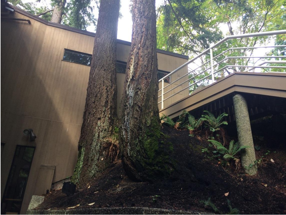
Tree #163 and #164 – Douglas-fir trees adjacent to the home in a small planter box
